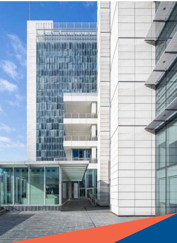
● GARIBALDI TOWERS - Milan
